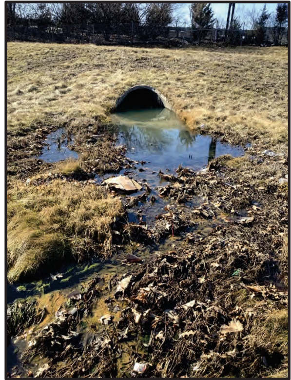
27. View of UNT 4 at existing culvert outlet, facing upstream west. 1/31/2024
