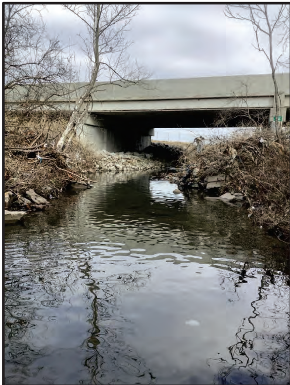
26. View of Coldwater Creek flowing underneath I-70 bridge, facing upstream south. 1/31/2024
