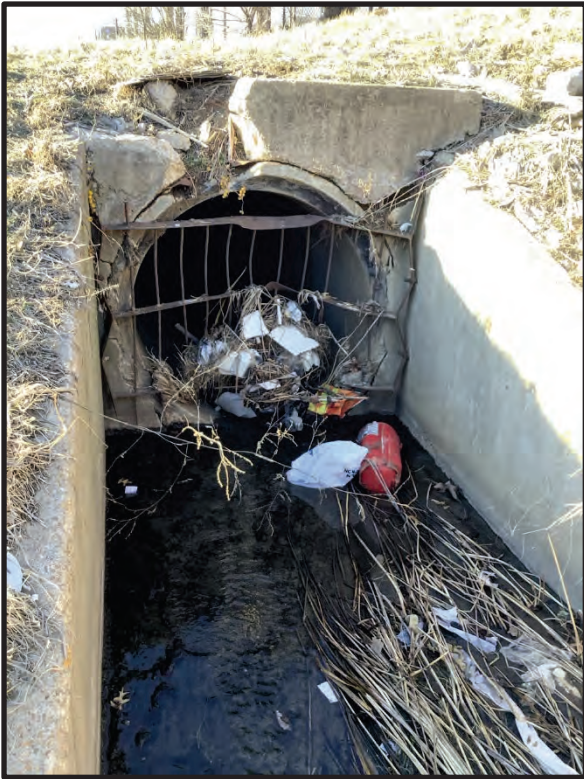
85. View of SF 12 at existing culvert outlet, facing west. 1/31/2024
