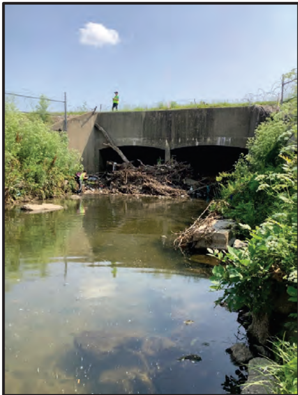
46. View of Coldwater Creek bridge, facing downstream northeast. 5/24/2023
