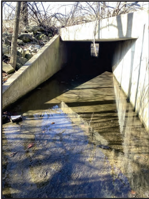
9. View of UNT 3 at existing box culvert outlet, facing upstream west. 1/31/2024
