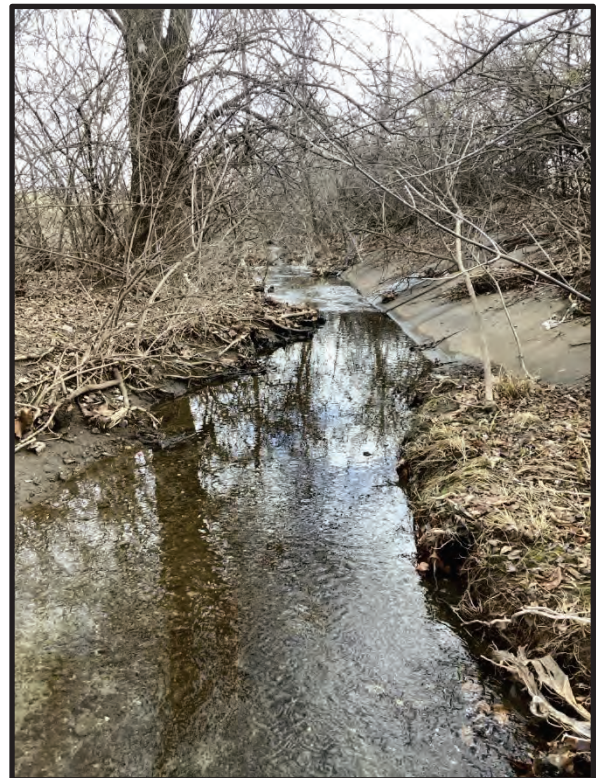
20. View of UNT 3 – Concrete Portion, facing upstream west. 1/31/2024
