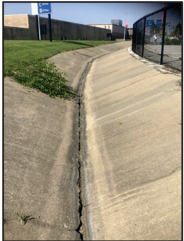
56. View of SF 9, facing northeast. 5/23/2023
