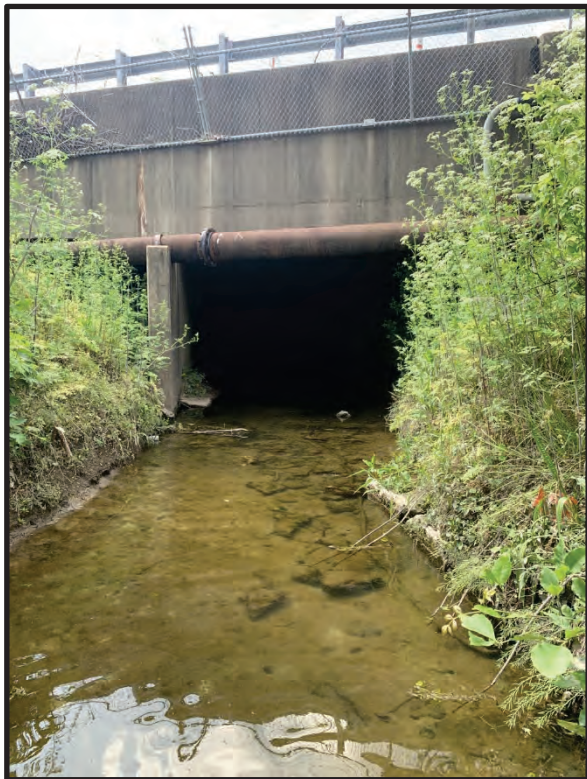
50. View of UNT 1 underneath existing box culvert, facing upstream northwest. 5/23/2023 5/24/2023
