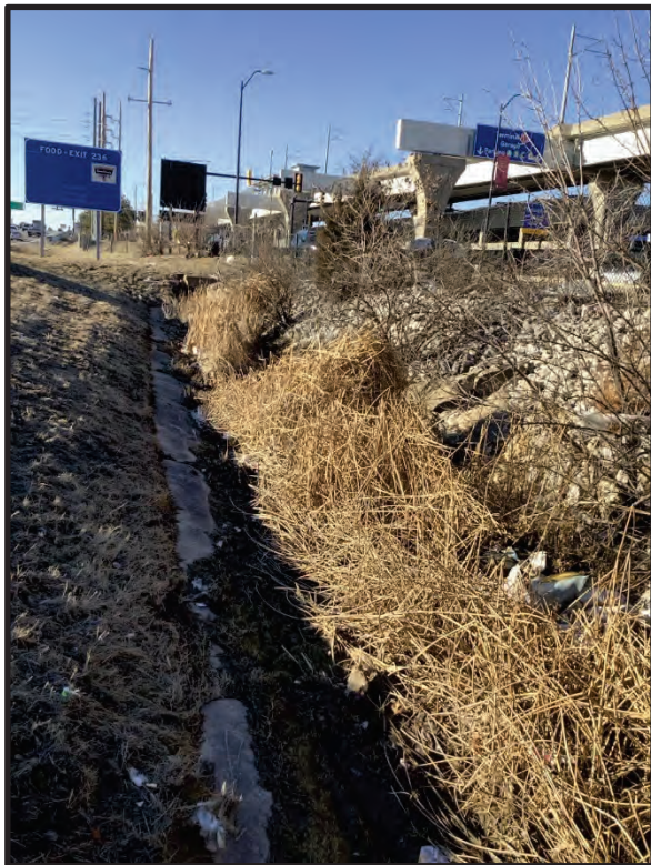
86. View of SF 12, facing northwest. 1/31/2024
