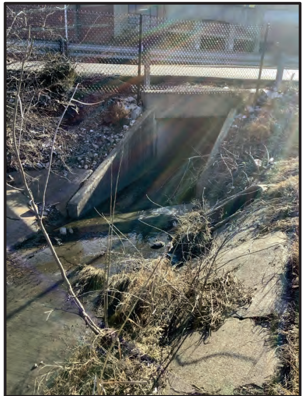
80. View of SF 11 at existing culvert outlet, facing southwest. 1/31/2024
