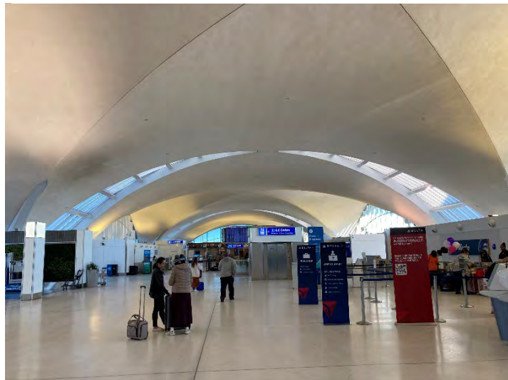
Figure 6: Terminal Building Historic Domes (Interior)
