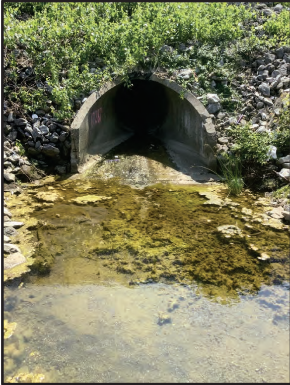
93. View of SF 14 at existing culvert outlet, facing south. 5/24/2023
