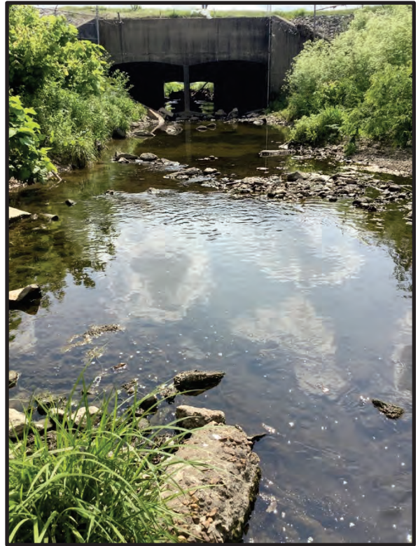
47. View of Coldwater Creek bridge, facing upstream southwest. 5/24/2023
