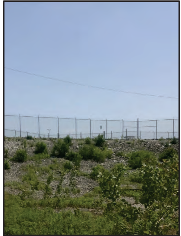
91. View of stormwater detention basin, facing north. 5/24/2023
