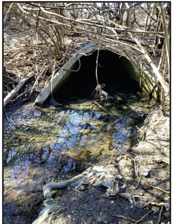
32. View of UNT 5 at existing culvert outlet, facing upstream west. 1/31/2024
