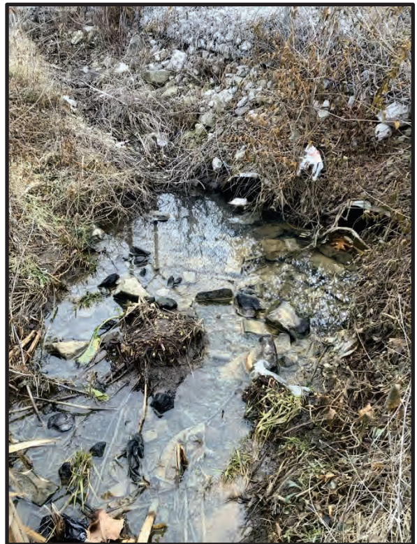
60. View of UNT 6 at existing culvert inlets, facing downstream southeast. 5/23/2023
