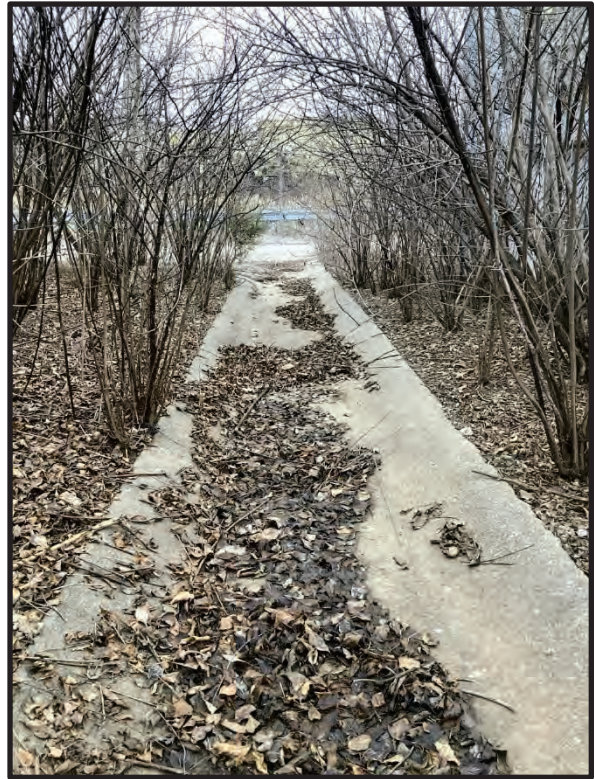
75. View of SF 10, facing northwest. 1/31/2024
