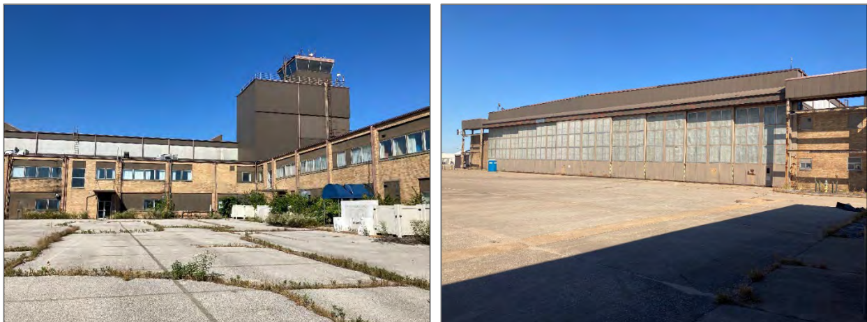
Figure 8: Existing MoANG Buildings (Lambert Field Historic District) to be Demolished
