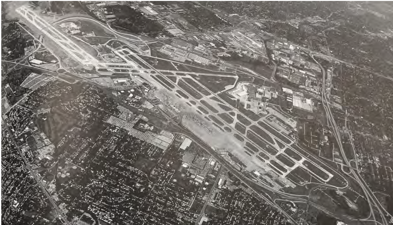
Figure 4-14: View of new Runway 11-29 under construction in 2005
