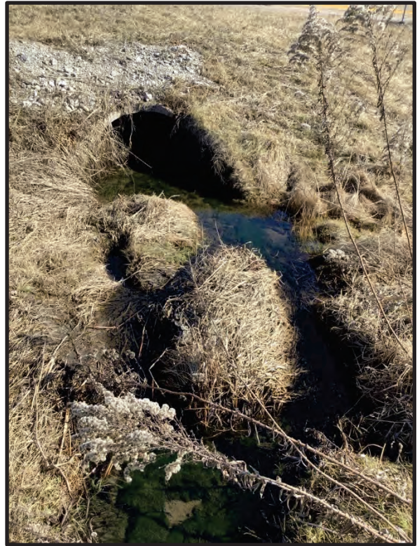
35. View of culvert inlet and UNT 5, facing downstream east. 1/31/2024
