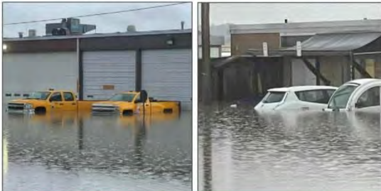
July 2022 Flooding at the Airfield Maintenance Facility
