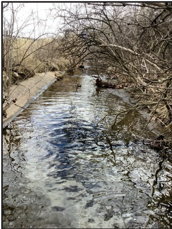
22. View of UNT 3 – Concrete Portion, facing downstream east. 1/31/2024
