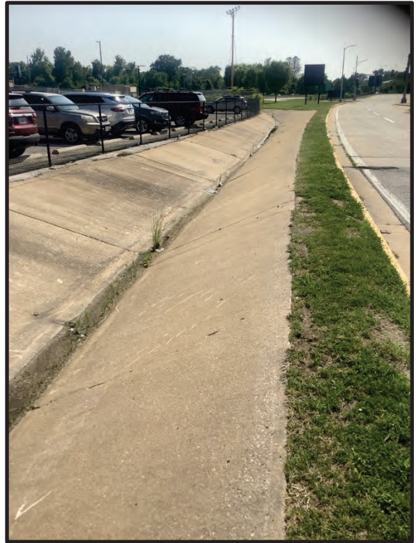
55. View of SF 9, facing southwest. 5/23/2023
