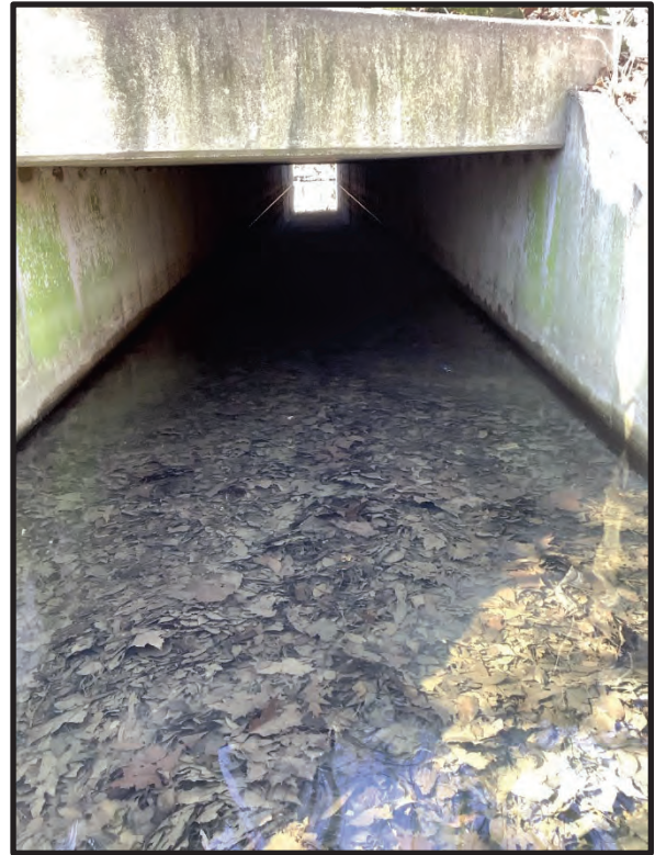
11. View of UNT 3 at existing box culvert outlet, facing upstream west. 1/31/2024
