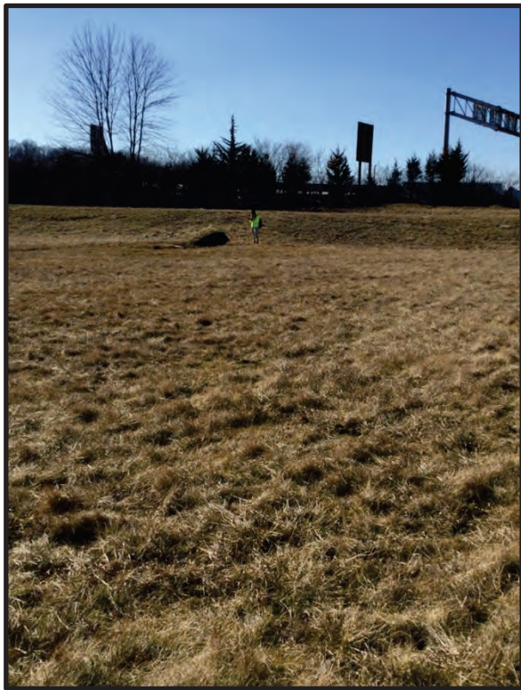
30. View of existing stormwater detention basin, facing southwest. 1/31/2024
