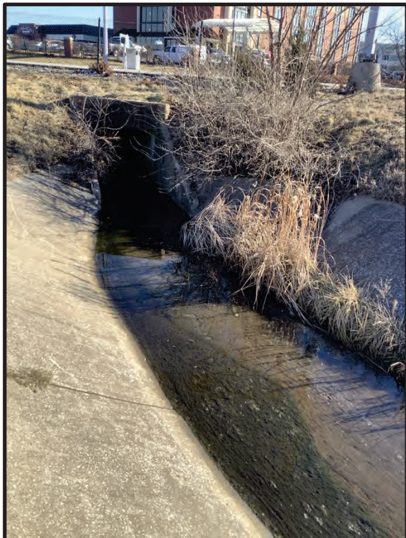
82. View of SF 11 at existing culvert inlet, facing southeast. 1/31/2024
