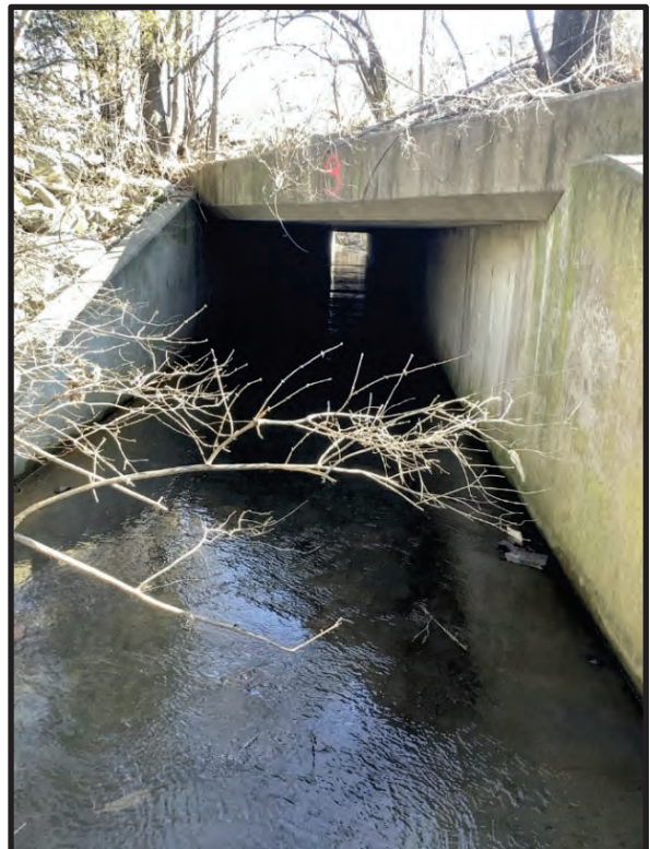
8. View of UNT 3 at existing box culvert inlet, facing downstream east. 1/31/2024
