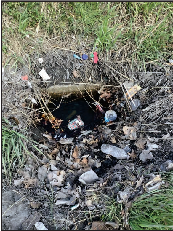
73. View of existing ground culvert inlet collecting water from SF 16. 3/20/2023
