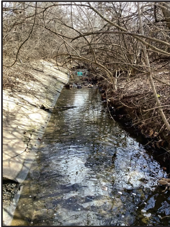
17. View of UNT 3 – Concrete Portion, facing downstream east. 1/31/2024
