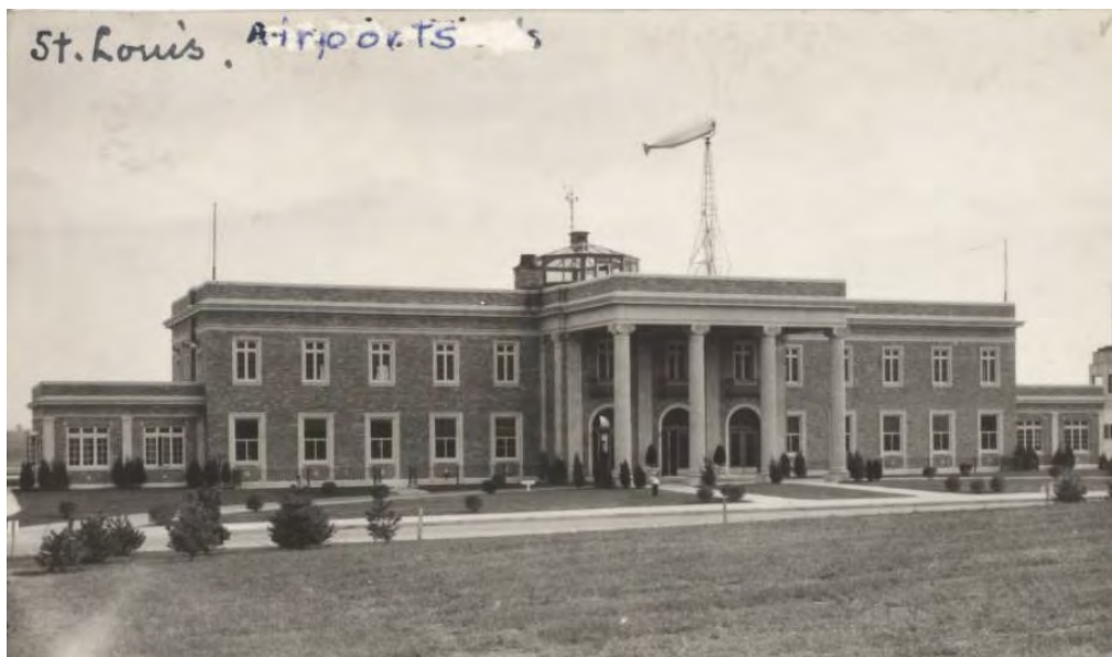
Figure 4-7: Photograph of Administration Building at Lambert Field, St. Louis. Postmarked 1935
