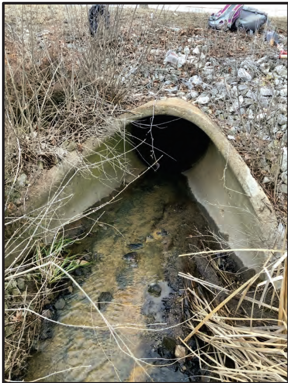
58. View of UNT 6 at existing culvert outlet, facing upstream northwest. 5/23/2023
