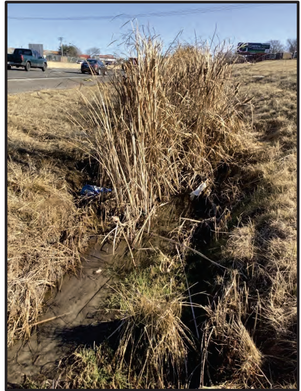
67. View of UNT 7, facing upstream southeast. 1/31/2024
