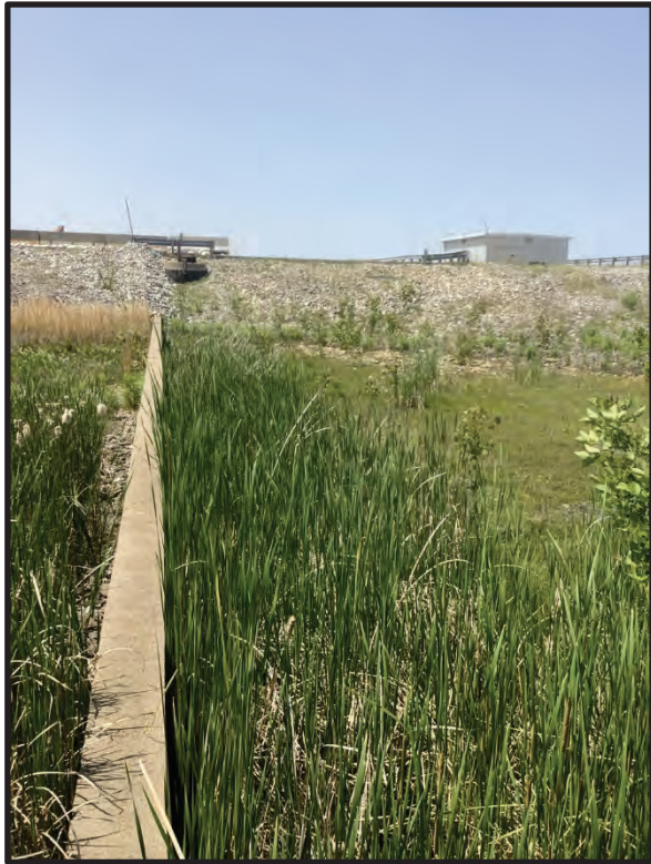
89. View of stormwater detention basin, facing north. 5/24/2023
