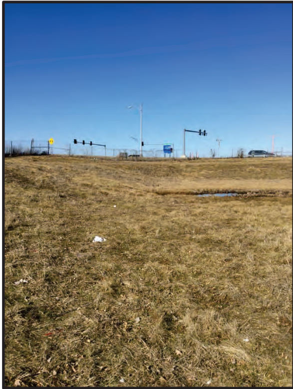
29. View of existing stormwater detention basin, facing northeast. 1/31/2024
